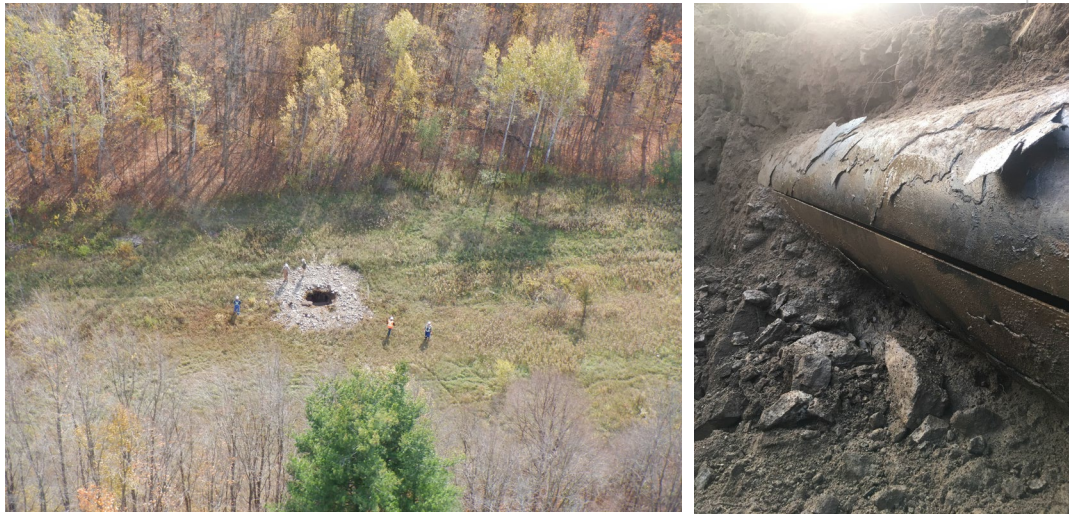
Figure 1: HydroTest failure location and ruptured pipe
