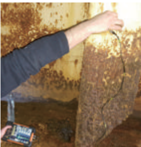
Port dock thickness measurement
