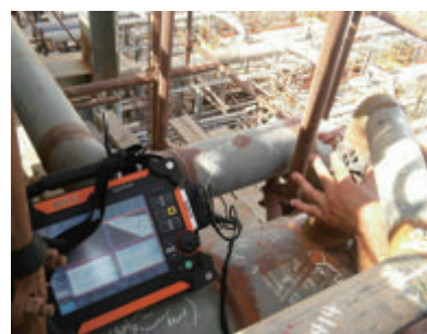
Tube weld inspection
