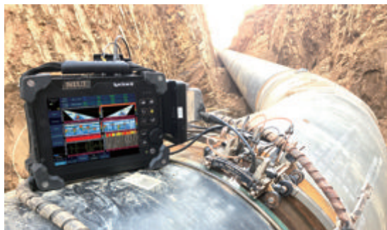
Pipe weld inspection
