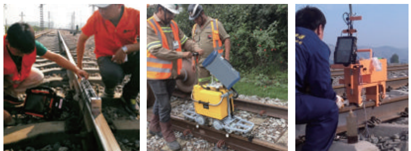
● PA testing for weld
